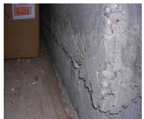
Repair work is often required to kicker before next lift can proceed.
