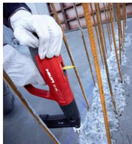
X-FS Form Stop being installed.
