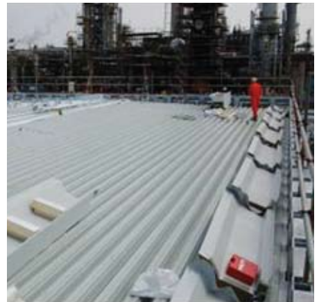
Liner Tray fixed to structural steel.
