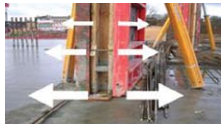
Outward pressure increases towards the bottom.
