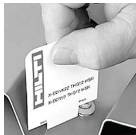
Checking the standoff of an X-EDNK22 roof deck fastening with a plastic template.
