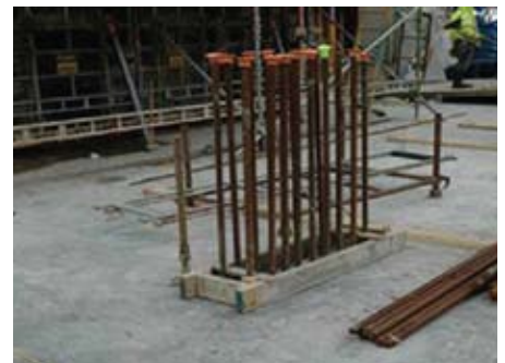
Kicker often build using old materials and concrete from the end of the last ‘pour’.
