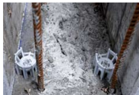
Form Stop locates inner face of form work.
