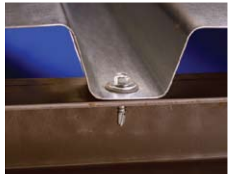
Liner Tray fixed to structural steel.
